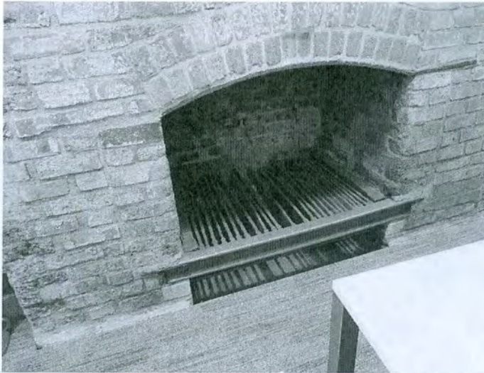
A former furnace on the river side of shed. Note the recycling old rails and
