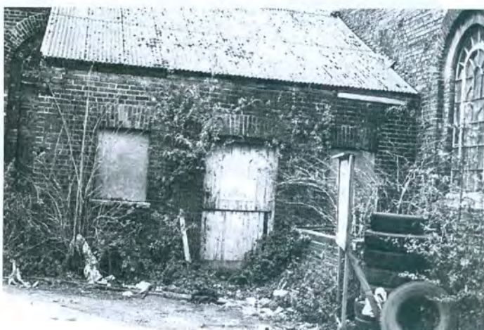
The former railway horse stables on south east side of the goods shed in 2008.
