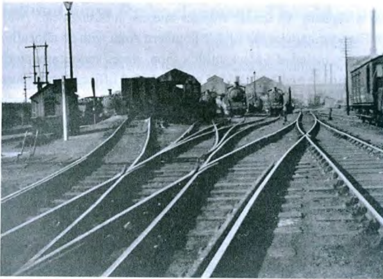
A ground level view from near the Black Bridge west to the Engine Shed yard including the coaling stage and east side of the shed with the goods shed in the distance. Photo Mr. Johnson c1935.
