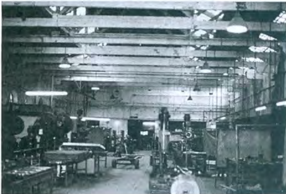
The interior of the south portion of the shed as occupied by Grill Floors Ltd in 1991. Note the original roof smoke vents and the rails in the floor. The view is to the west wall.
