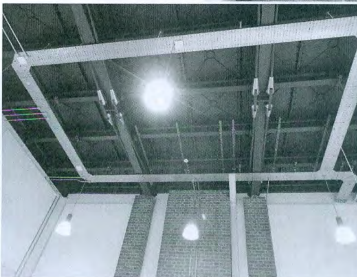
The underside of the water tank.
