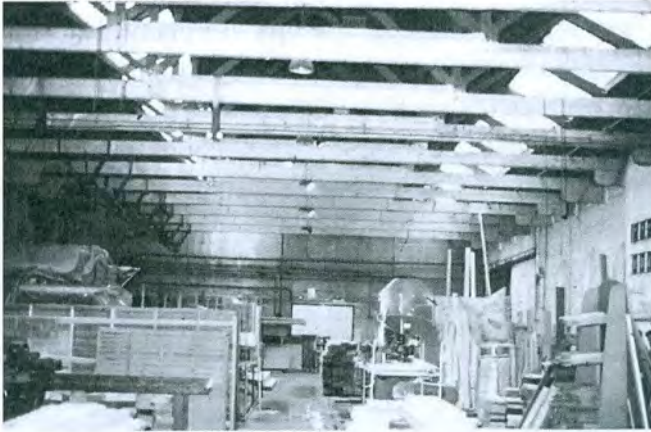
A general view of the County Timber Supplies side of the shed in 1991. It is probably the stacked timbers that hid further original features.
