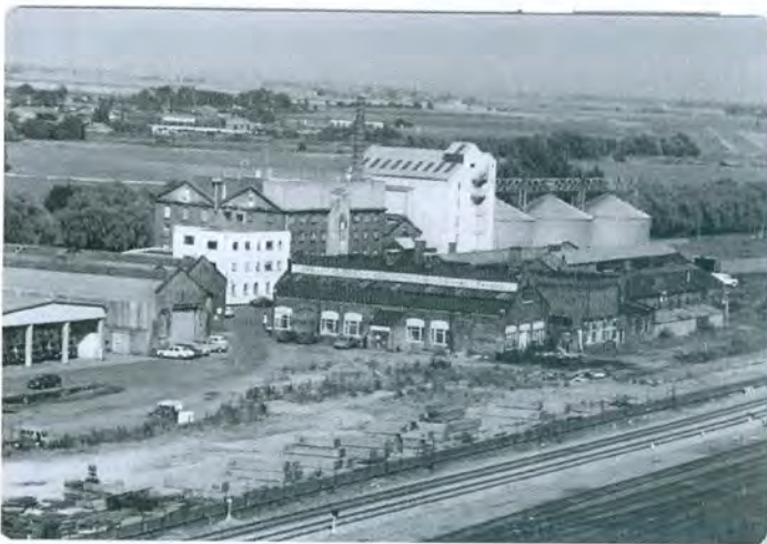
The former Peterborough East Station and sheds on 11 th August 1981 as viewed from the top of Apex House on the corner of Oundle Road/London Road. The timber (centre) is stacked on the former platforms. Left is the old Goods Sheds and centre the former engine shed with the workshop in front. Note the Grill Floors Ltd sign. Beyond are the Cadge & Colman flour mill, river Nene and the Embankment.
