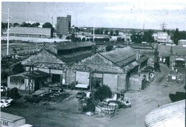
The engine shed in 1992 from the roof of the Mill grain silo. Note the marked sag in the south side roof. The Cadge & Colman weighbridge and mess room are by the north wall. Note also the top of the two water tanks.
